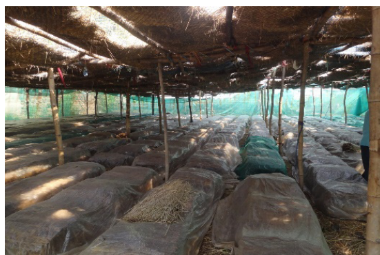
B. Temporary shed
